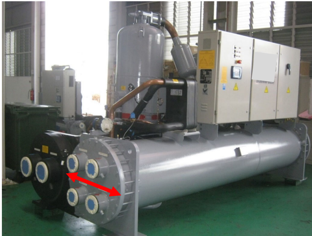
Primary Chiller with Double Bundle Condenser
